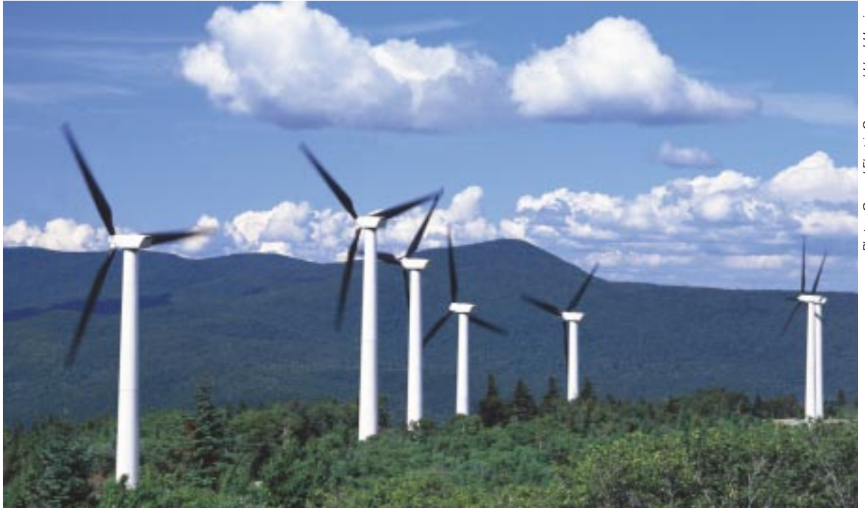
Photos: General Electric Company / Lloyd Herziger
